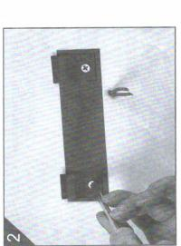
Use two screws to secure the lamp holder to the wall
